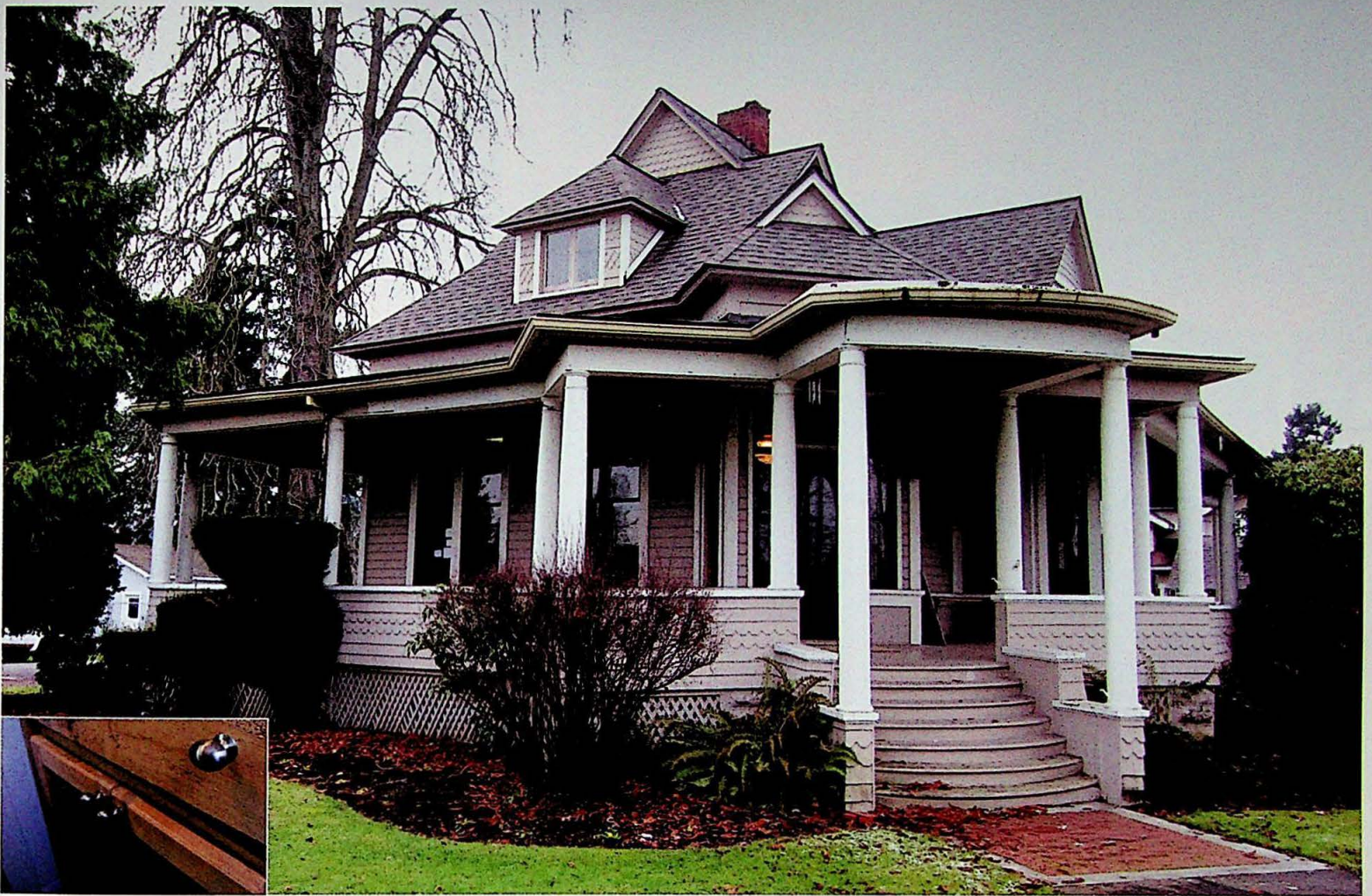
HOME FRONT Above: The John Meeker House doesn't look much different today than it did in 1890. Newspaperman Robert Montgomery enlarged the porch in the early '30s. Inset: One of the cabinets Dick made out of maple boards he found stored on the property.
