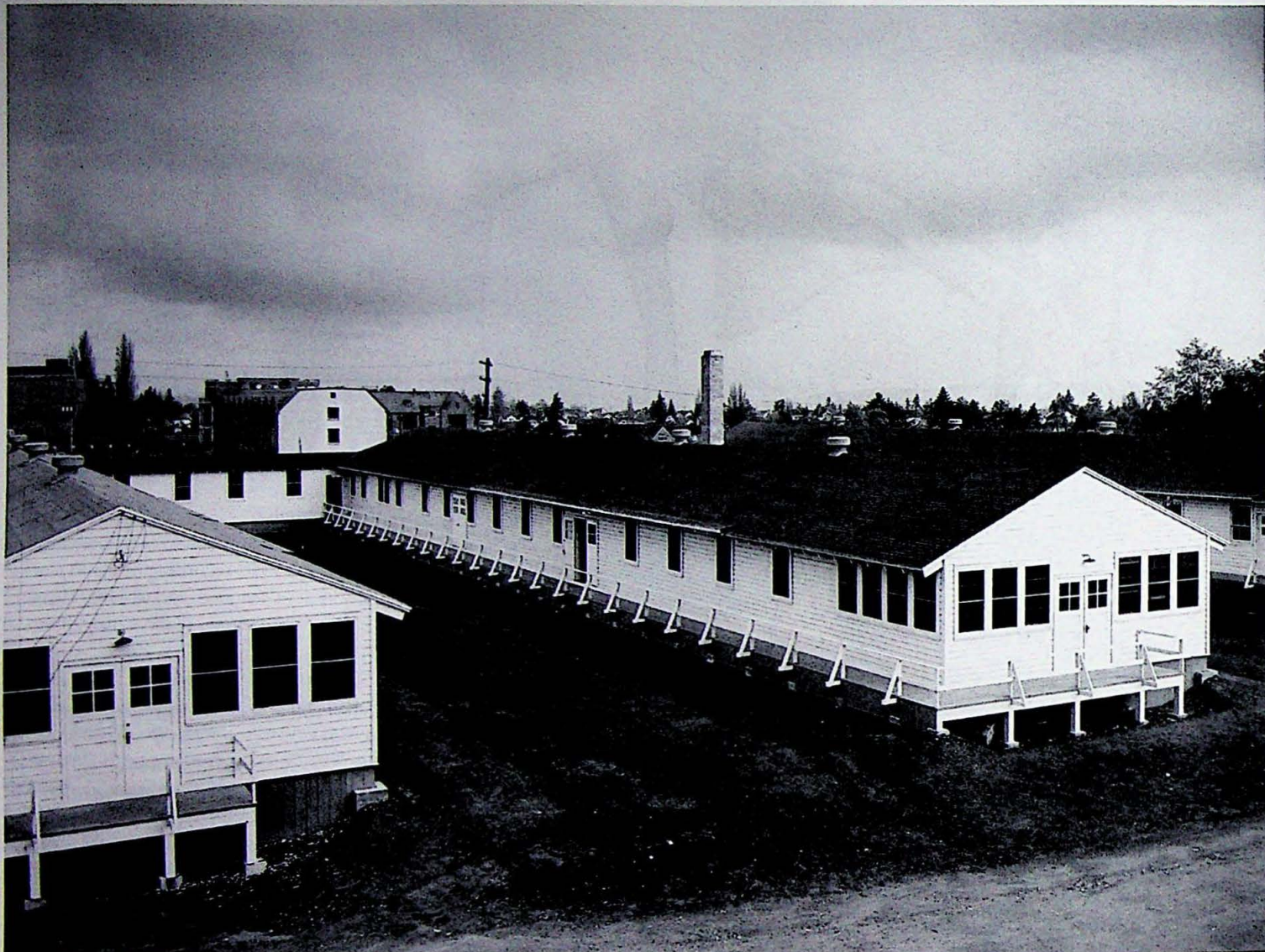
RECYCLED The war-surplus hospital buildings that would become known as South Hall were moved from Paine Field in Everett and reassembled in parade order on campus in 1947. Beyond them, Todd Hall, which was nearing completion when this photo was taken in late '47, can be seen.
